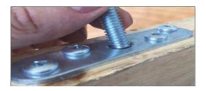
**9**. Center the second mounting plate on the bottom of the pivoting door with the flat side facing out. Using the starter holes, screw it in place with 32-mm (1-1/4-in.) no. 10 screws.
