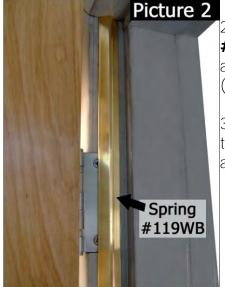
2. Next install the **acoustic seal Spring #119WB** on the jamb, on the side of the hinges, approximately 1/2 in (13 mm) from the doorstop. (Picture #2)
