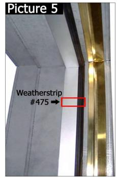
Now install the acoustic seals on the two jambs. Then attach the Snap-On Covers (technical drawing) before installing the acoustic seal on the head
